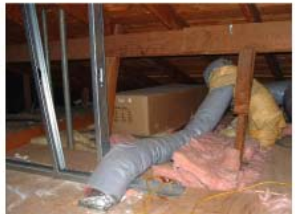
NW Corner of Attic
