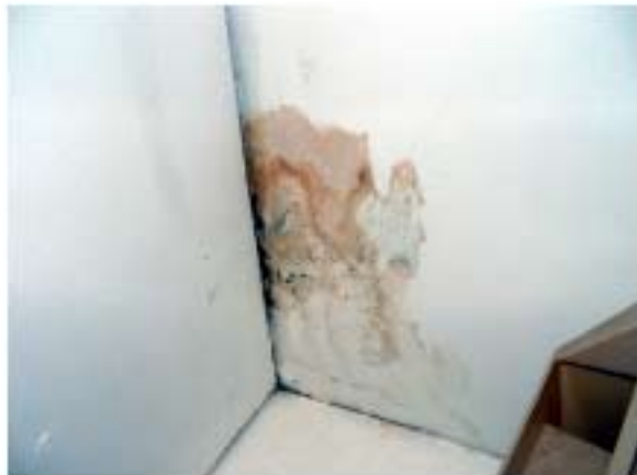
North Wall Behind Dresser
