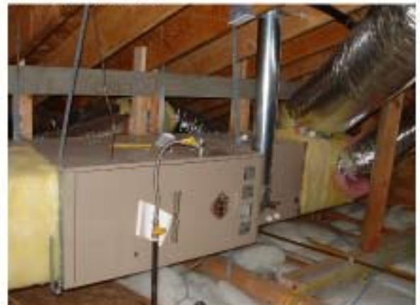
SW Corner of Attic
