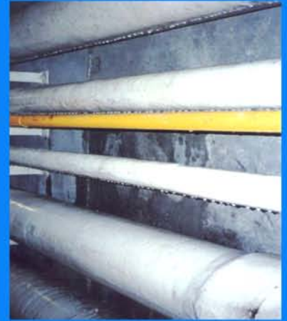
After Anabec Advanced Cleaning Solution
